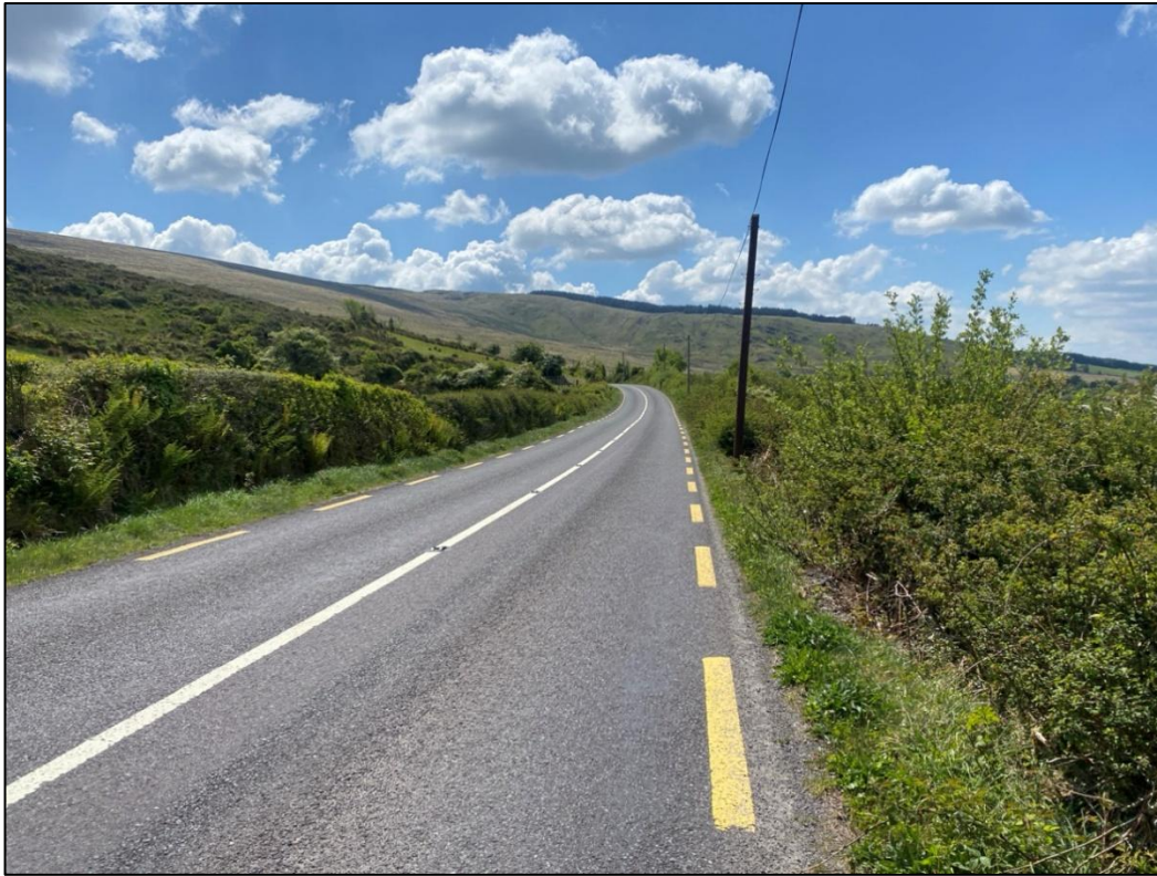
Plate 6-34 Existing Road network where the Proposed Grid Connection will be installed classified as Buildings & Artificial Surfaces (BL3) .
