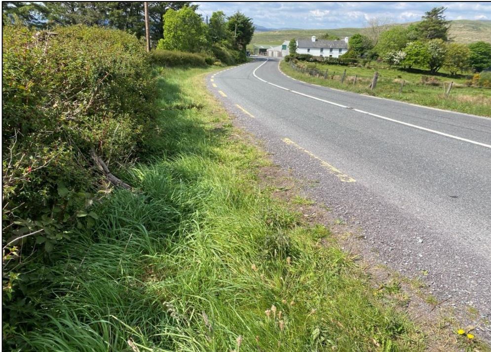
Plate 6-22 Public Road located to the centre of the Proposed Wind Farm classified as Buildings and Artificial Surfaces (BL3) .
